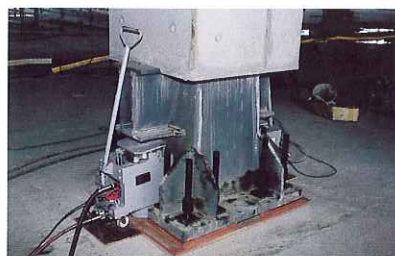
ターミナルビル柱脚 Jacking up a pillar of the Passenger Terminal Building
