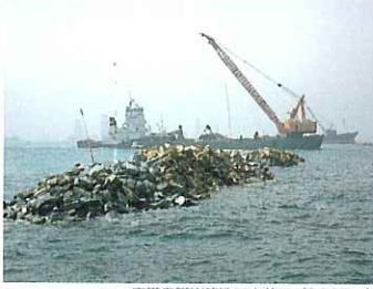
空港島護岸築造工事着工(1987.1) Start of the airport island seawall construction (Jan. 1987)
